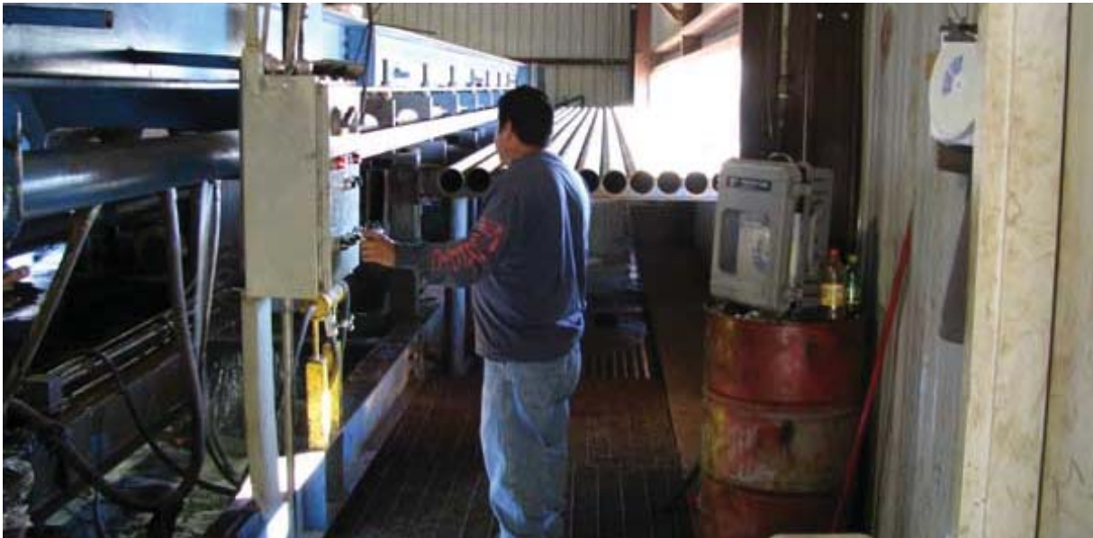
picture 6: Hydrostatic Test
